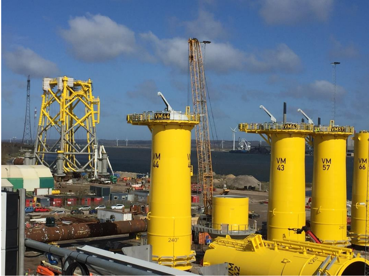
Transition pieces awaiting transport onto an offshore windfarm's site. (c) Sandbag 2016
